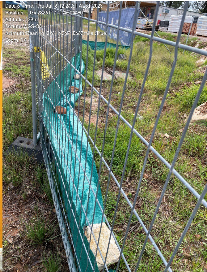
Sediment fence around contractor parking area.
