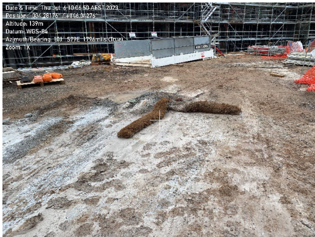
Concrete wash / spillage.
