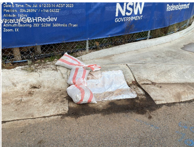
Geotextile pit filter sediment trap.
