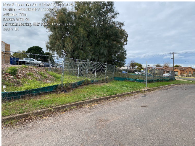
Sediment fence around contractor parking area.
