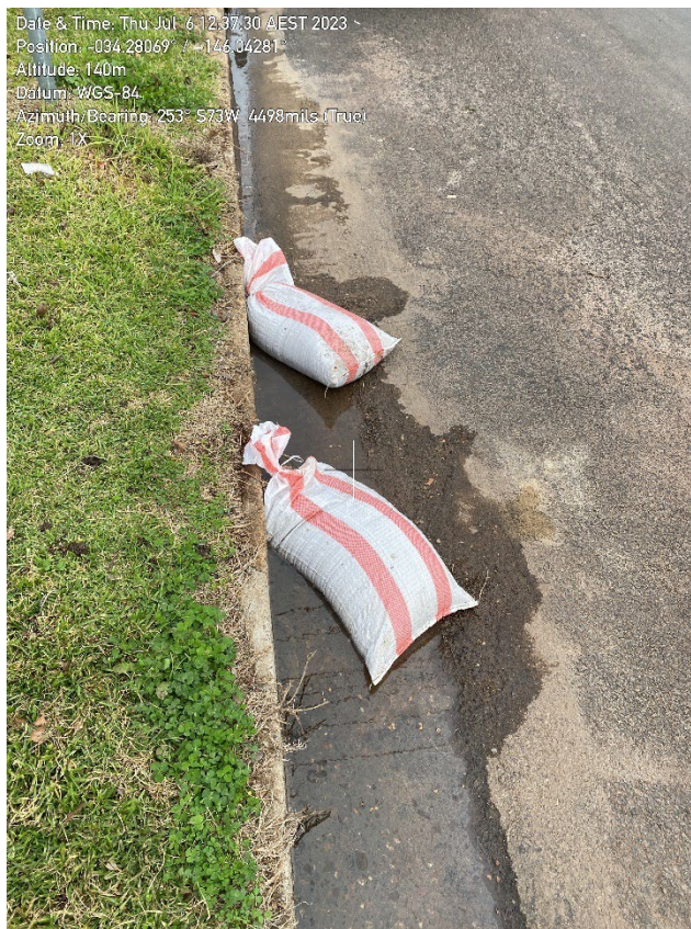
Check dams in gutter upgradient from the site entrance.
