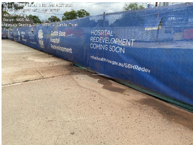
Sedimentation on footpath down-gradient of the project site. Green sediment fence seen behind blue hoarding.
