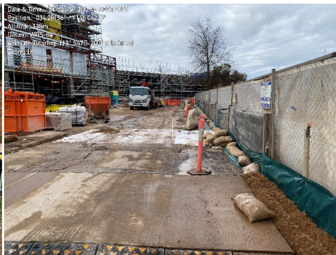
Sediment fence, coir logs and sand bags as a sediment control and to secure the base of the sediment fence.
