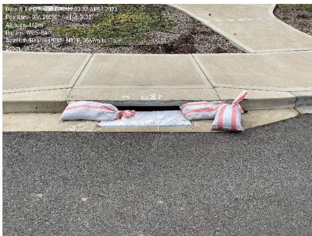
Geotextile pit filter sediment trap in accordance with ESCP.
