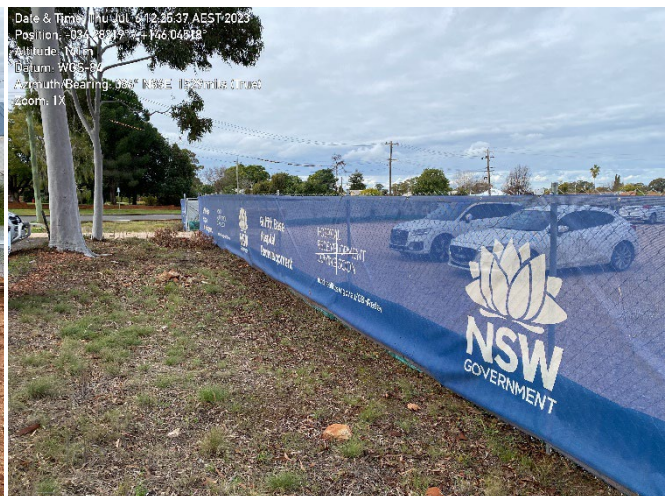
Sediment fence and hoarding for contractor parking.
