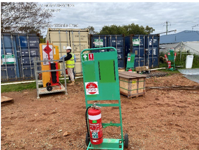
Dry chemical fire extinguishers around flammable cabinet.
