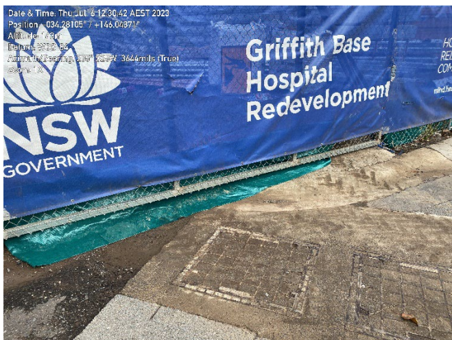
Sediment fence unsecured along gate.
