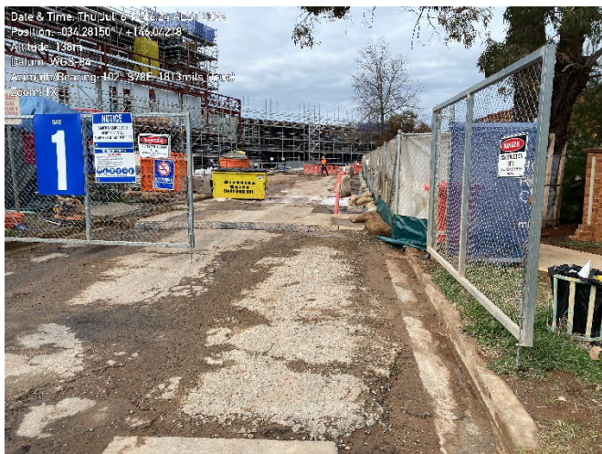
White geofabric is changed weekly to remove sediment deposition from vehicles trafficking across the rumble grid (when in place). Riverina skip bin for waste management.
