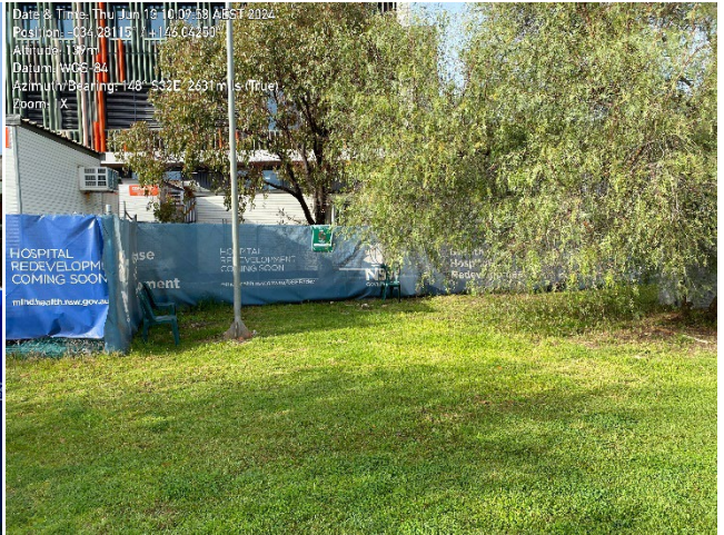
Tree protection in place.
