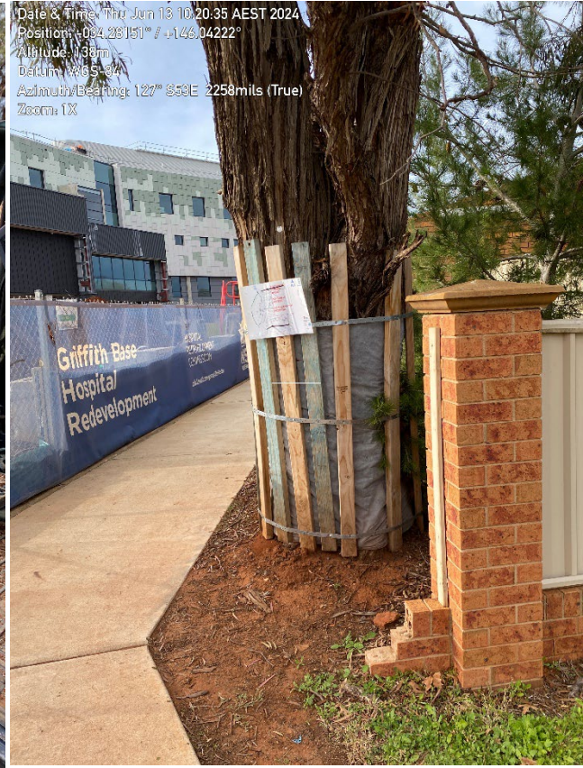
Tree protection. No sediment visible on the path beyond the southern boundary.
