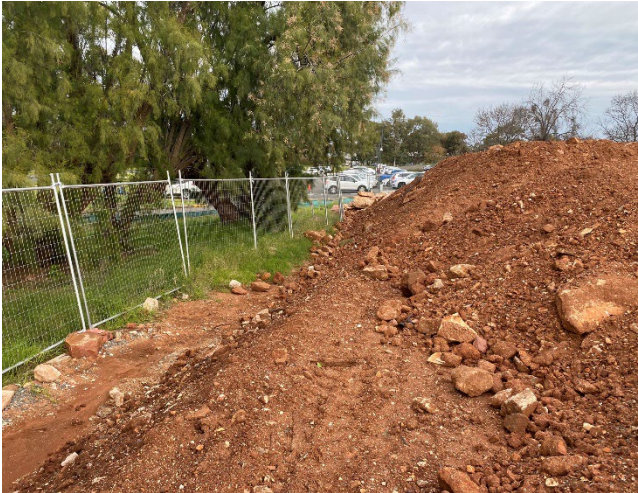
Soil stockpile in contractor parking compound.
