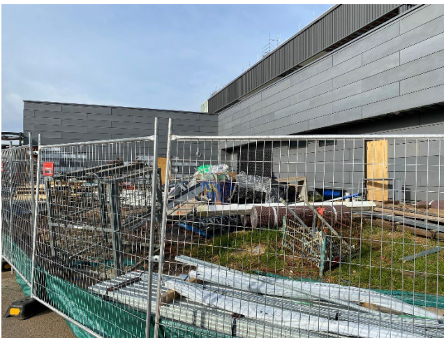
Construction storage, sediment fence along north-western boundary of the site.
