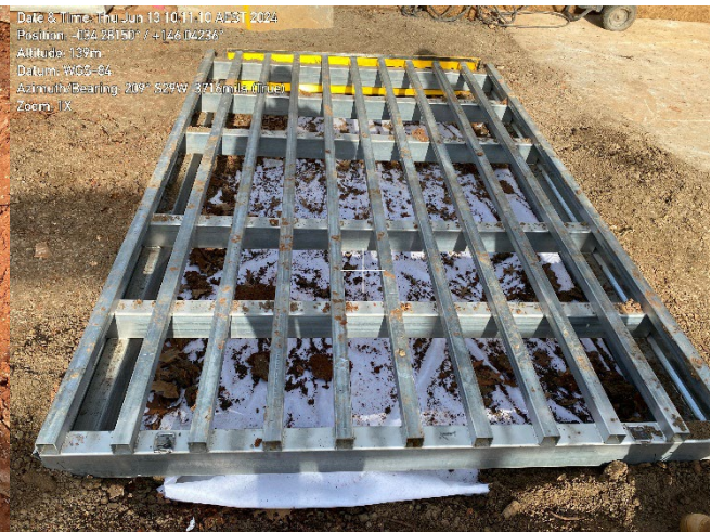
Construction site access with geotextile under rumble grid.
