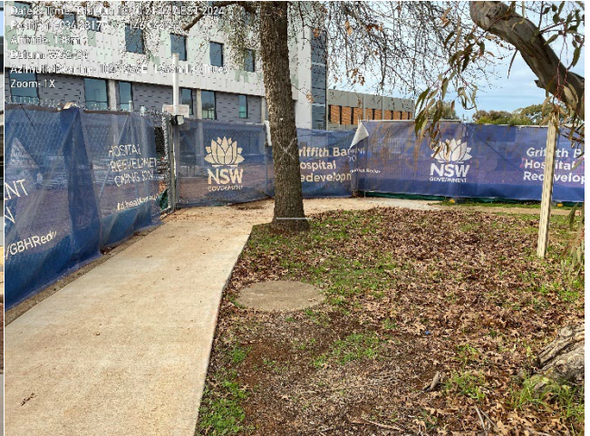
Sediment-free footpath down-gradient of the project site, along the southern boundary.
