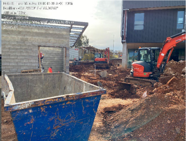
Area undergoing earthworks for retaining wall in proximity to south-western boundary.
