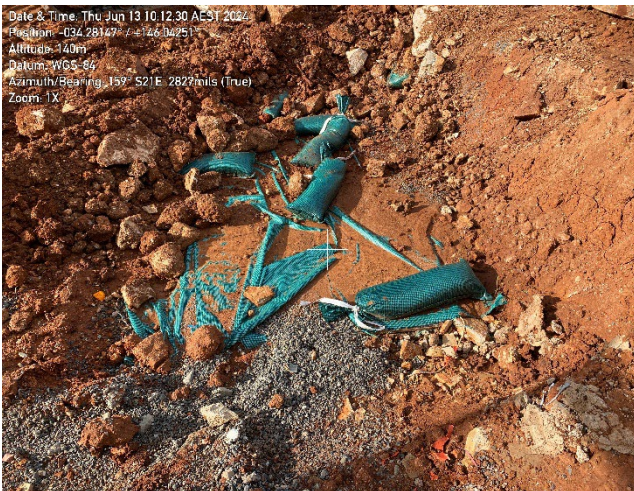
Covered stormwater drain that is not currently operational.
