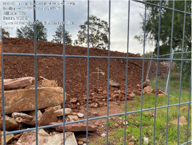
Soil stockpile at contractor parking within 3 m drip line of trees.
