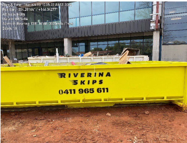
Skip bins on site.
