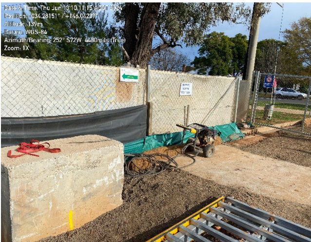
Sediment fencing along the southern Project boundary.
