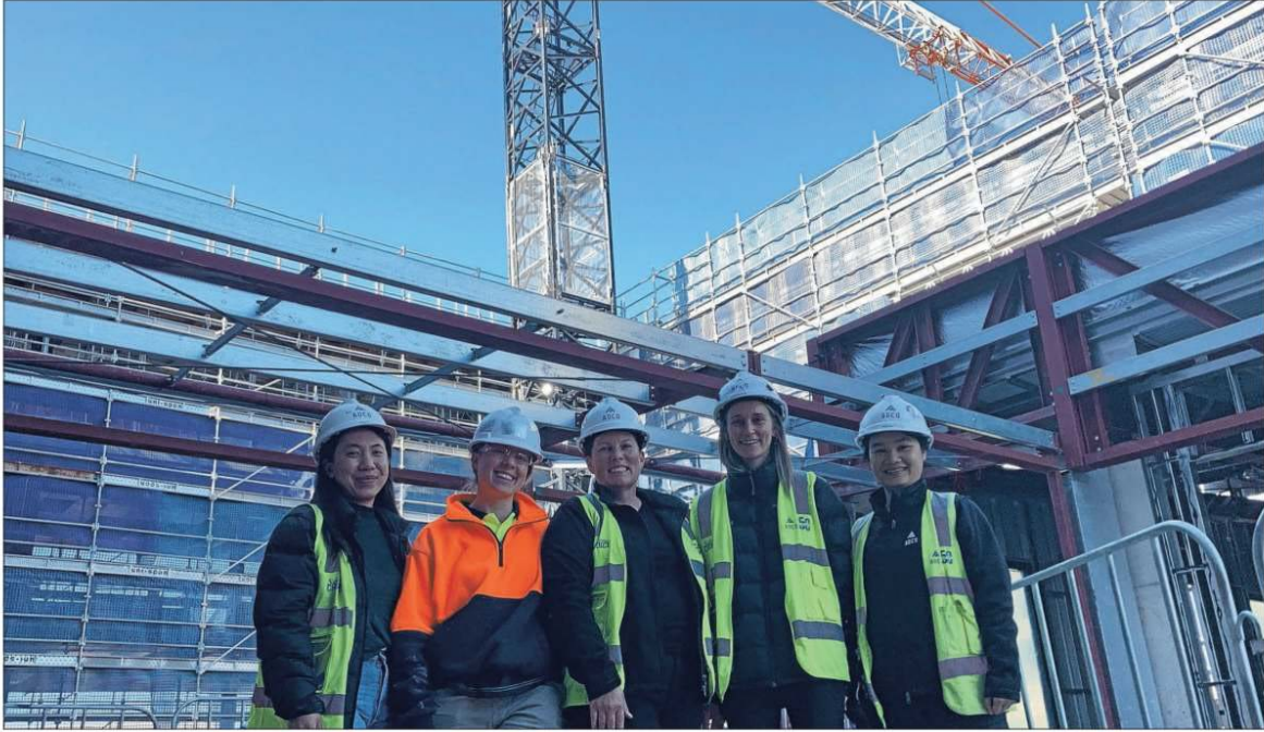
Erica Drummond, Maria Gallinger, Gemma Irvin, Eliza Blight and Shallmae Lao are hard at work on the Griffith Base Hospital redevelopment. Picture by Cai Holroyd
