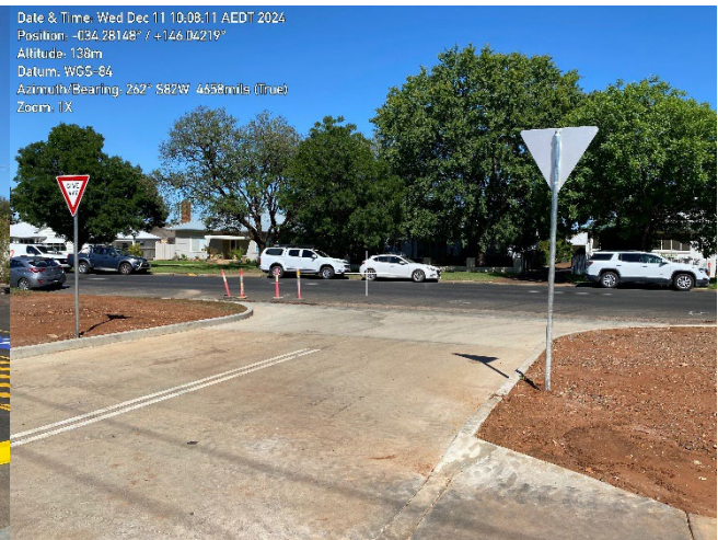
Photo 18 – entrance to hospital carpark and signage.
