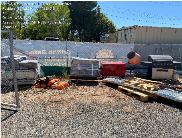
Photo 21 – material storage in site compound. Generally litter free.
