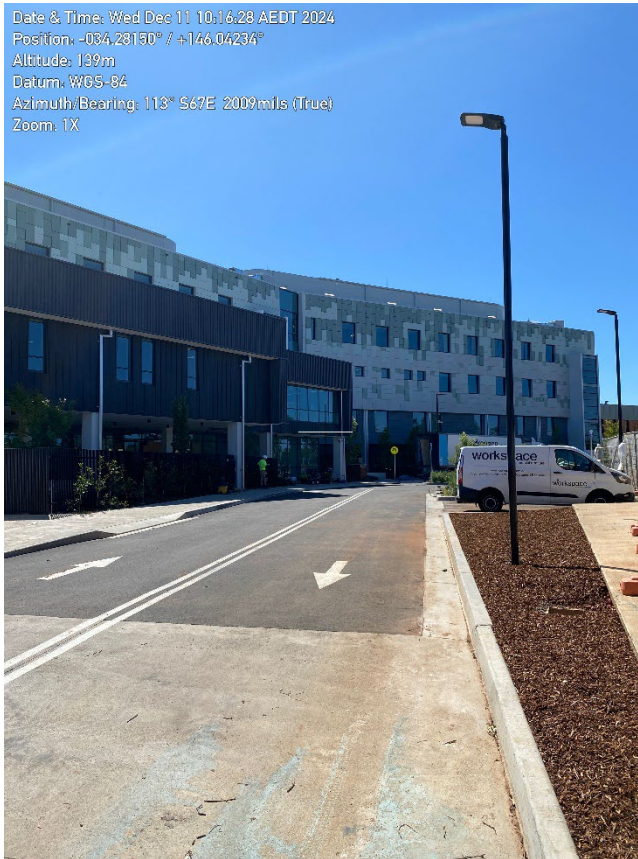
Photo 1 – sealed access, carpark and landscaping of Stage 1
