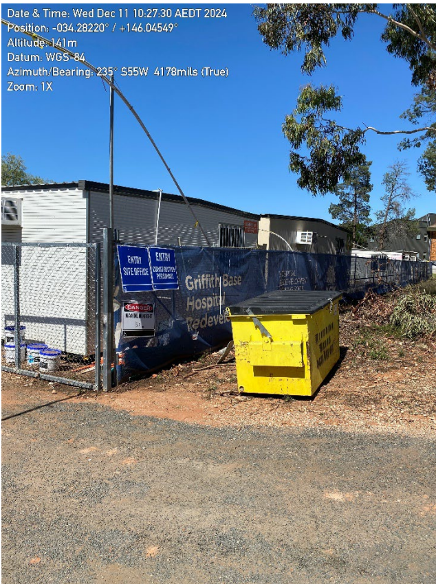
Photo 13 – Signage and hoarding at site compound entrance with waste skip.
