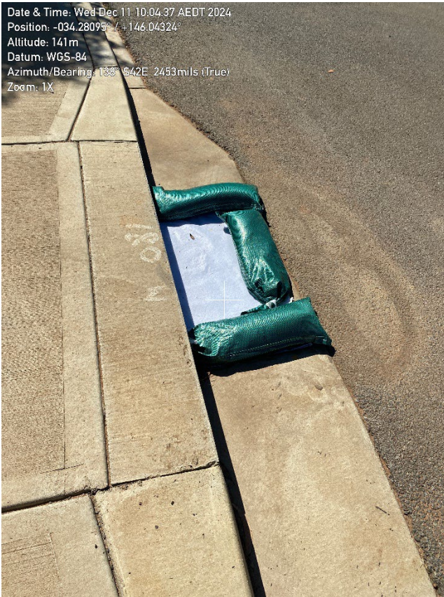
Photo 15 – geotextile and sandbags over drain as sediment control on Animoo Avenue.
