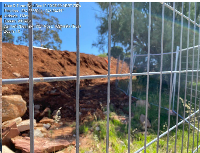
Photo 24 – toe of soil stockpile has been scraped back away from drip line of adjacent trees.
