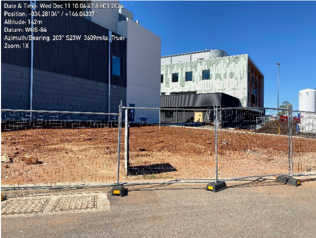
Photo 5 – exposed batters currently being topsoiled and seeded.
