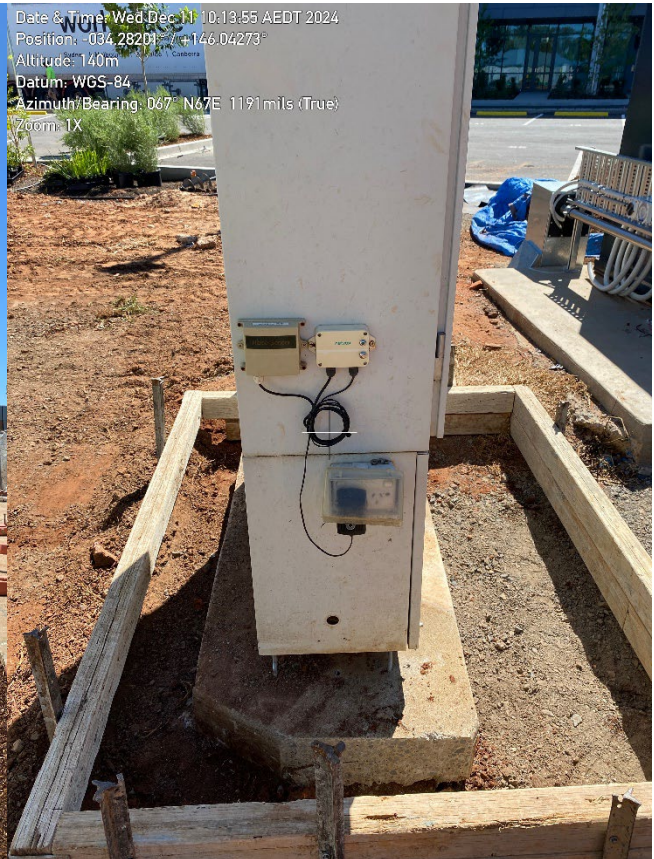
Photo 2 – example of noise sensor adjacent to south-eastern boundary.
