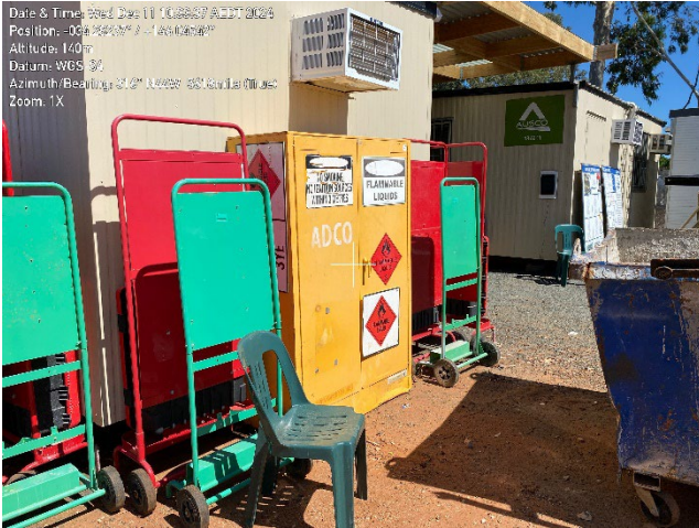
Photo 11 - Bundled and signed Flammable Liquids cabinet.
