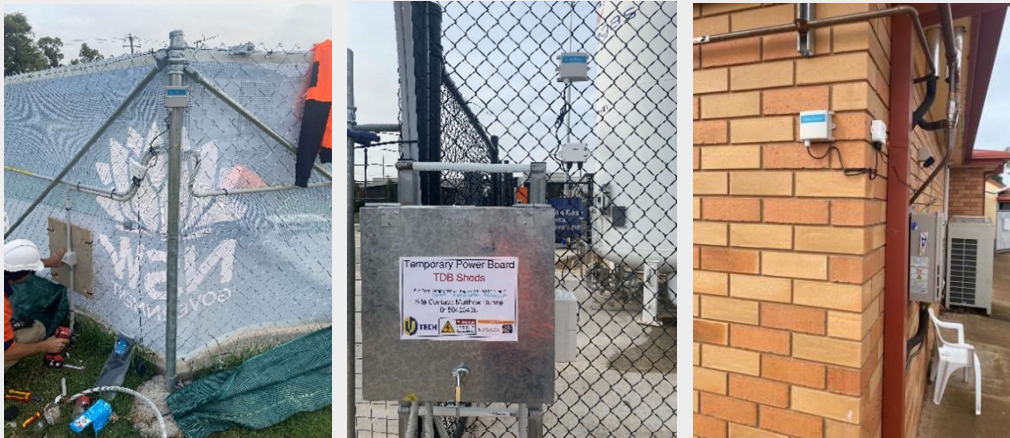
Fig 5, 6 & 7 show the locations of noise monitors NOISAU-009, 008 & 005 on site.
